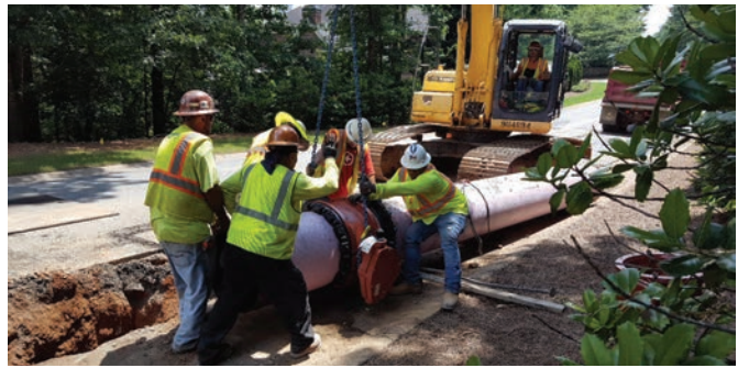
24-inch DI pipe is installed in Johns Creek, Georgia.
