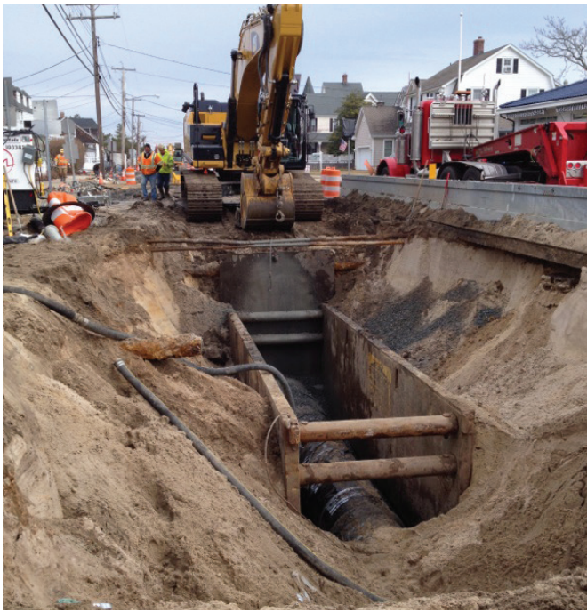
20-inch DI pipe is installed in Bay Head, New Jersey.
