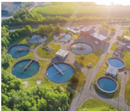
For water utilities, emphasis should be placed on energy savings when selecting pipe materials. Image Source: iStock
