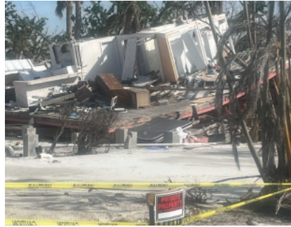
Hurricane Ian damage
