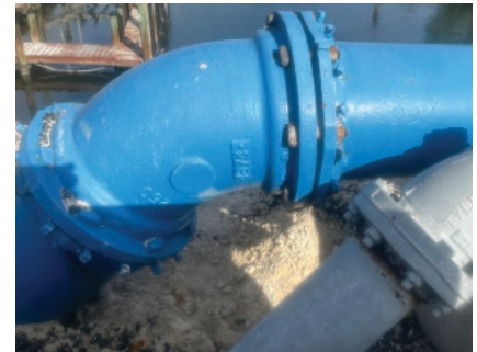
Hurricane Ian did not affect Ductile Iron piping on Sanibel Island. Notice the fitting cast in 1974!
