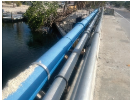
Hurricane Ian did not affect Ductile Iron piping on Sanibel Island. Notice the fitting cast in 1974!
