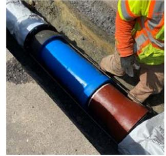
According to Bert Weiss, the city's field crew found the McWane Ductile ERDIP system "simple and easy to install." V-Bio® Enhanced Polyethylene Encasement was used on the retrofit, as it is a recommended laying practice listed in the ISO 16134 Standard, reducing friction on the pipeline by over 30%.
