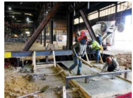
Floor is poured for two new high-speed casting machines.
