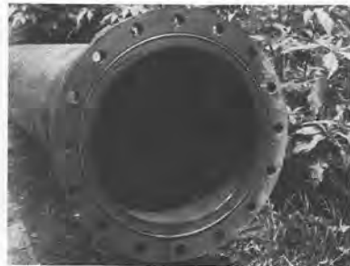
Flanged Joint, showing Gasket in groove
