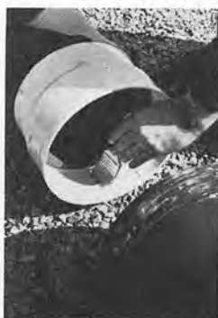
2. Apply Clow lubricant to the joint surfaces.
