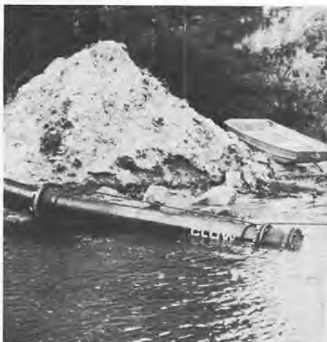
Installing Clow River Crossing Pipe by pulling it into position.
