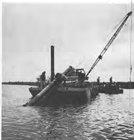
Installing Clow River Crossing Pipe by laying it from a barge.
