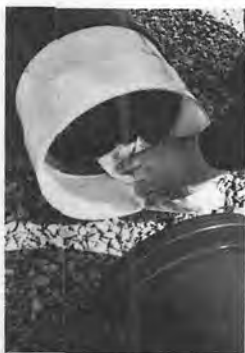
1. Wipe the surfaces of the joint clean.
