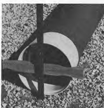
3. Push the spigot end into the "bell" until home.
