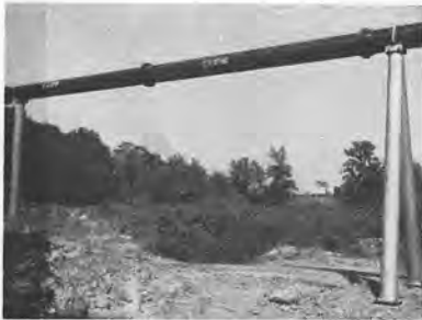
Installation of Clow Long Span Pipe
