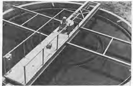
Typical installation of Yeoflo Clarifier in Municipal Treatment Plant
