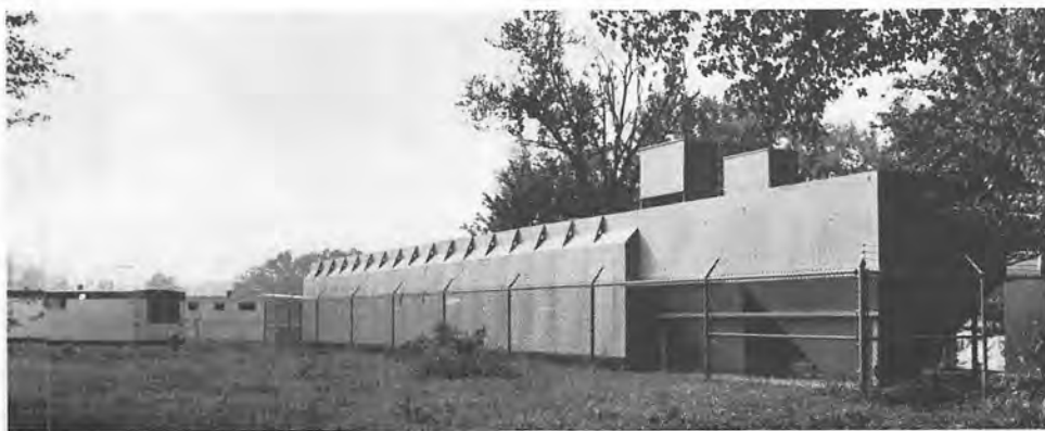
Mobile Home Park system—100,000 GPD capacity
